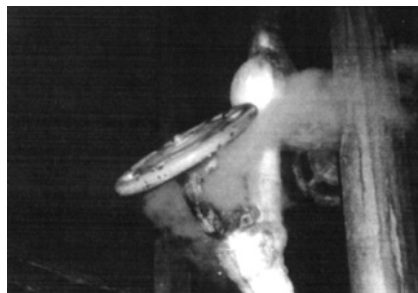
Continual stem leaks from globe valves allows plant efficiency to decrease and maintenance costs to rise.
