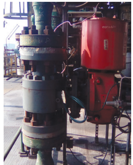
Above: One of several MOGAS 6-inch, ASME 2500 Class C-Series valve sits atop a coke drum in a South American refinery's water cutting application. This industry-proven valve is engineered specifically to perform in slurry and high erosion conditions.
