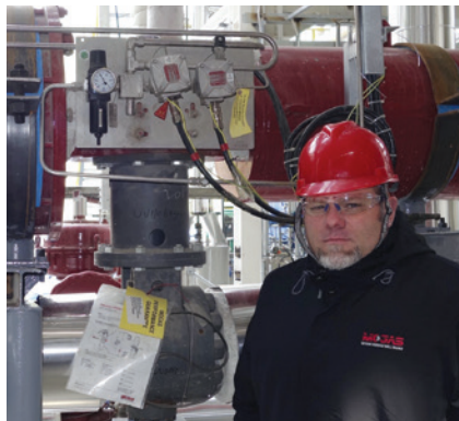
Above: One of several MOGAS 6-inch, ASME 2500 Class C-Series valve sits atop a coke drum in a South American refinery's water cutting application. This industry-proven valve is engineered specifically to perform in slurry and high erosion conditions.
